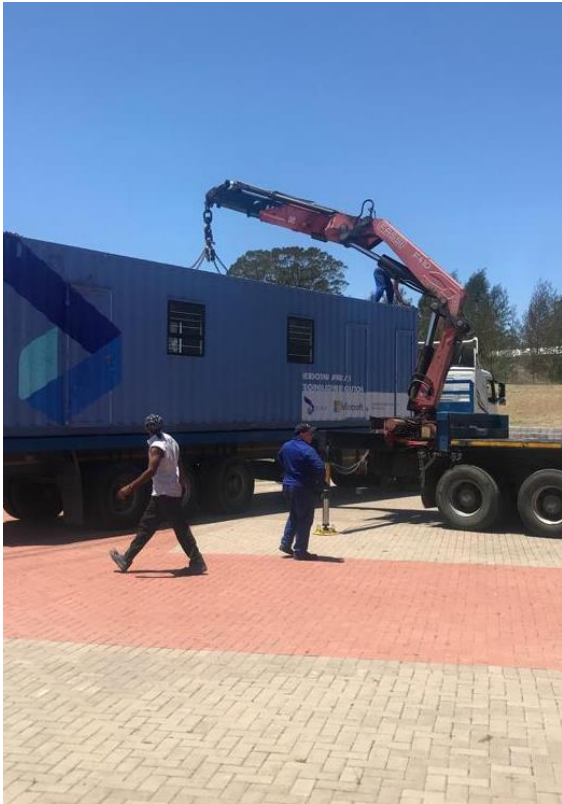
Setting up of off-grid digital mobile classrooms
